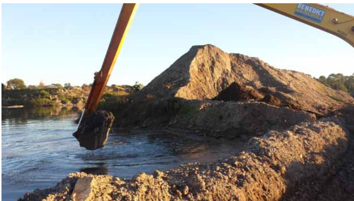
Photograph 4.2 Stockpile at the eastern end of the marina site, adjacent to the dredge pond
